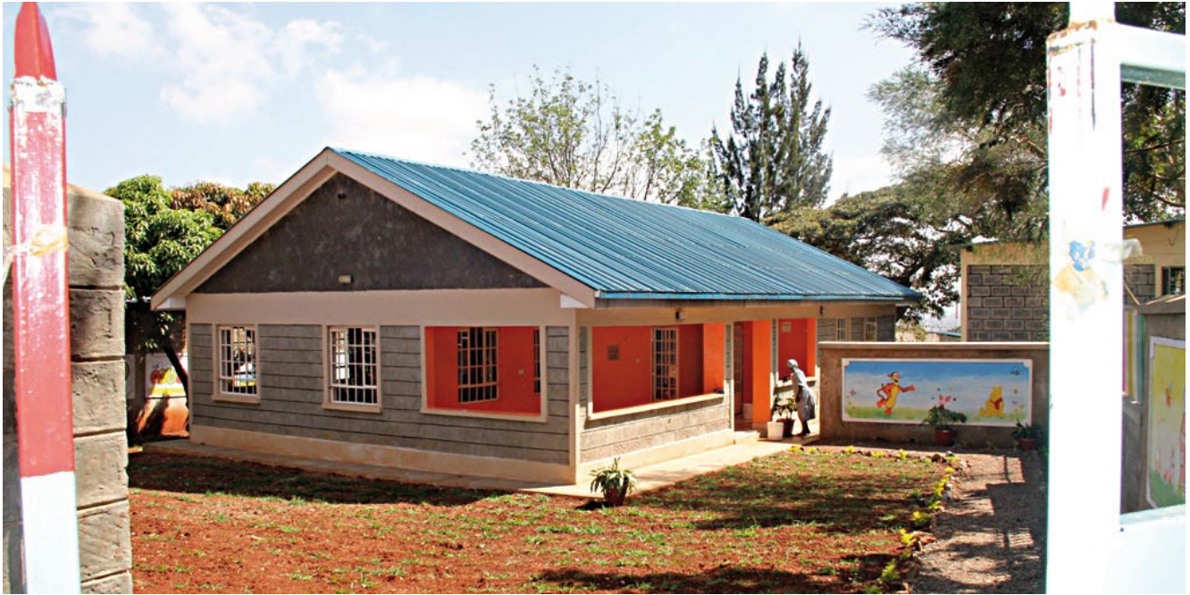
The Newly Built Child Care Center at Langata Women's Prison
